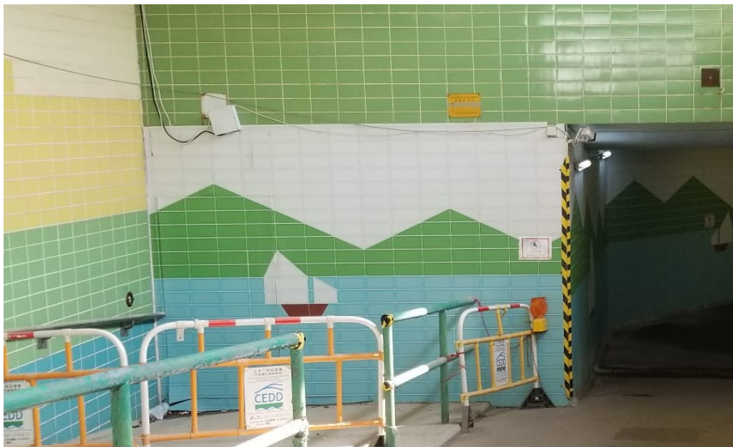
Photo 3 – Erection of site hoardings in unobtrusive colours
