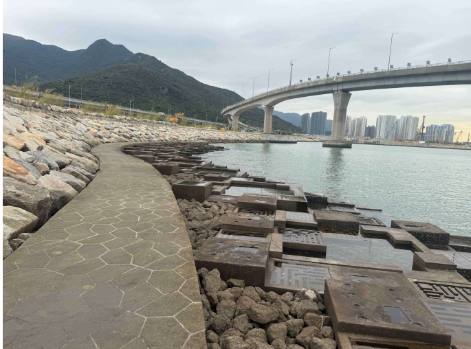
General View of Rocky Eco-shoreline
